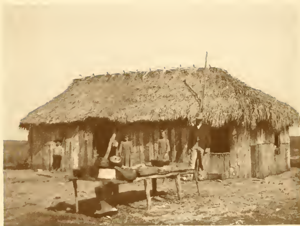
A trapper's home in the Everglades. The cabin is built of cypress bark and palmetto leaves
